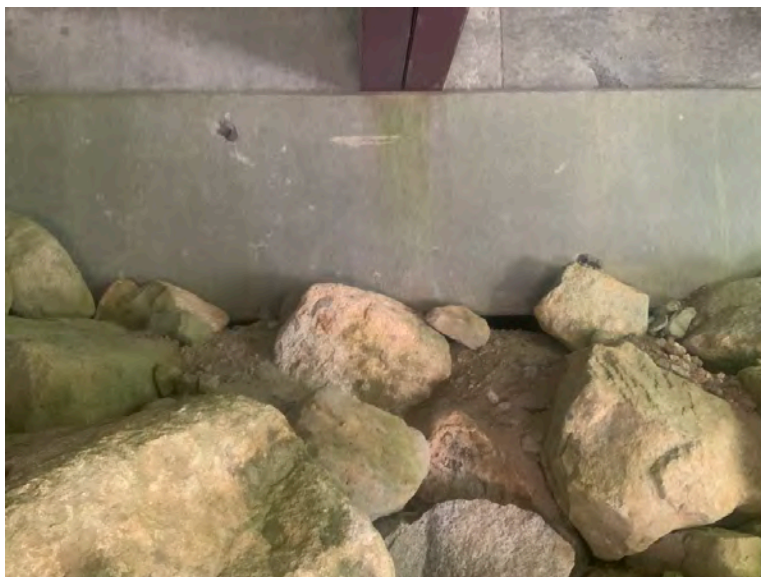
Left Bank Abutment when facing downstream
