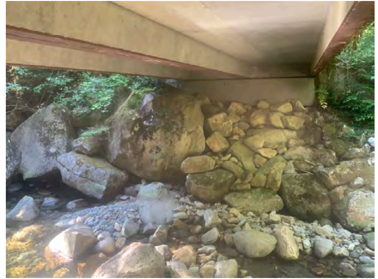
Left Bank Abutment when facing downstream
