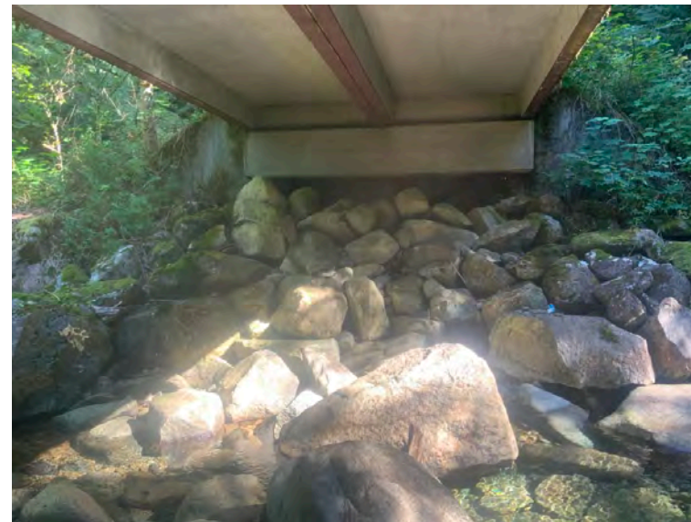
Right Bank Abutment when facing downstream
